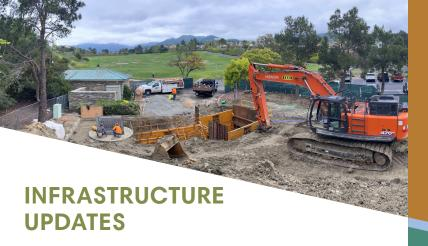
The District's largest ongoing capital project, the rehabilitation of the Golf Club Sewer Lift Station, is over 50% complete. A second phase will begin in early July and focus on upgrading mechanical components like pumps and valves — work which will require a complete bypass of the station. The entire project will be completed by early October 2024.
