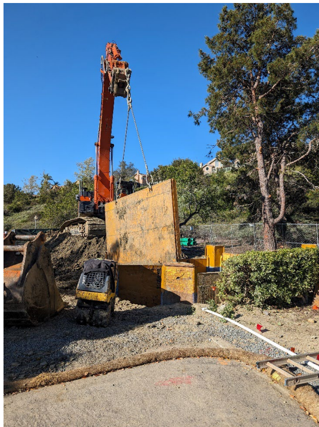
“Slide Rail Shoring” system being removed as backfill reaches grade.
