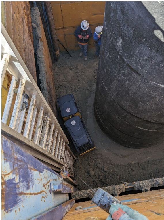
PHC utilizing a remote controlled, vibratory, sheep-foot roller.
