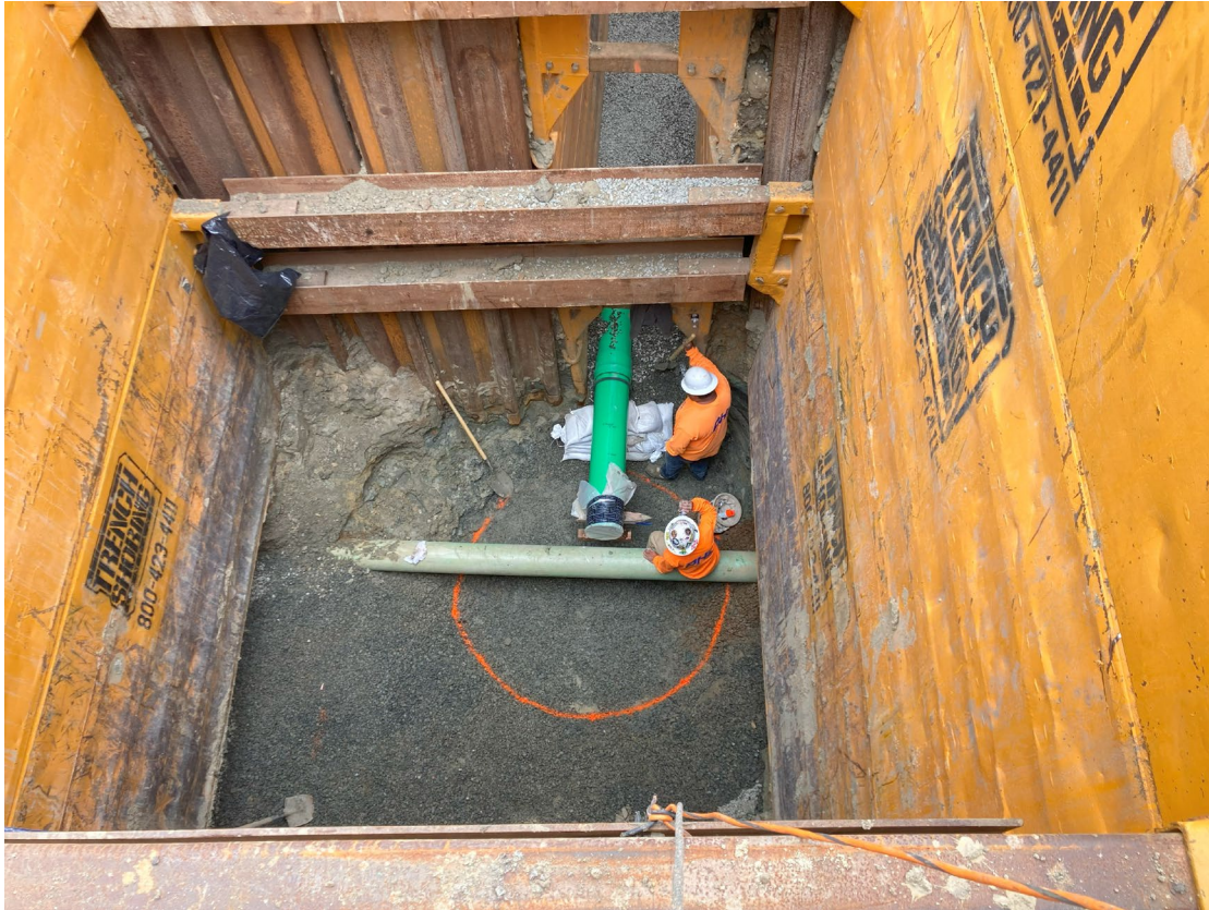
Bottom of Diversion Manhole excavation with 12-inch PVC Gravity Pipeline penetration.
