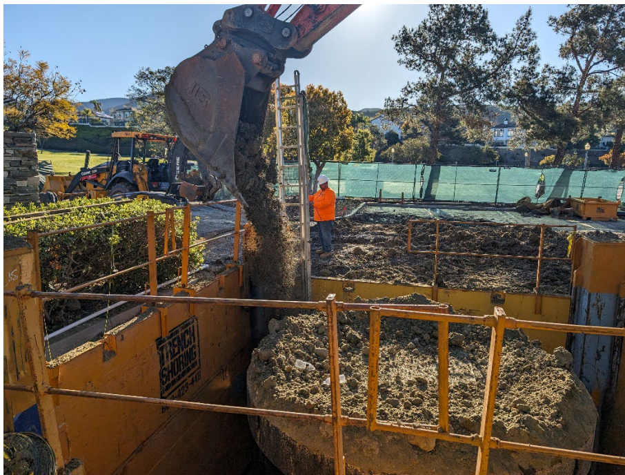
Native, backfill material being placed in Bypass Wet Well excavation.
