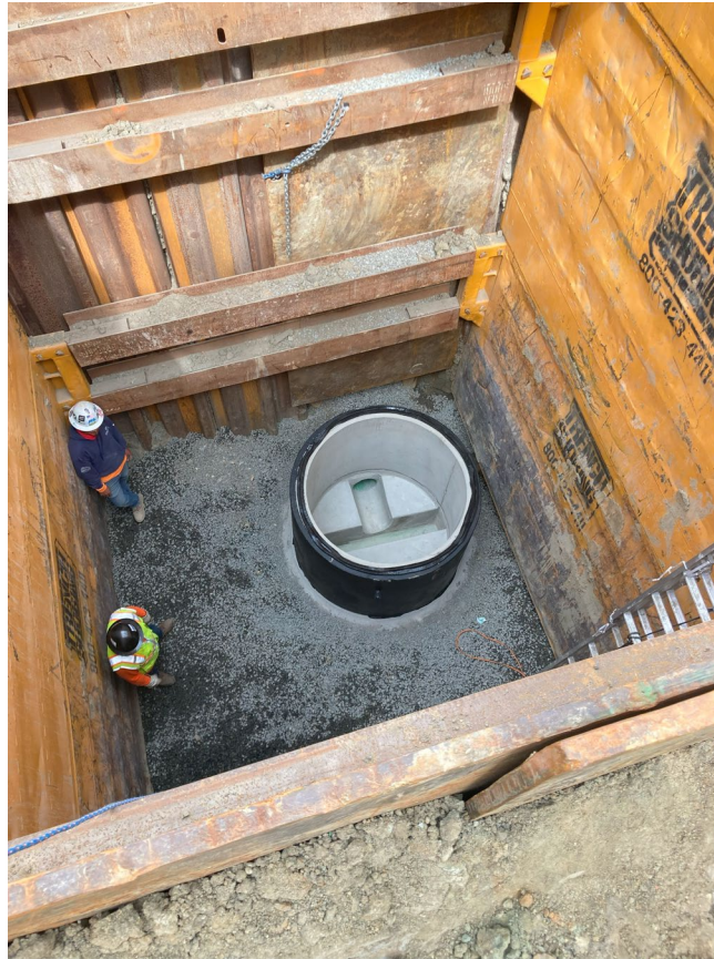
Delivery and install of Diversion Manhole.
