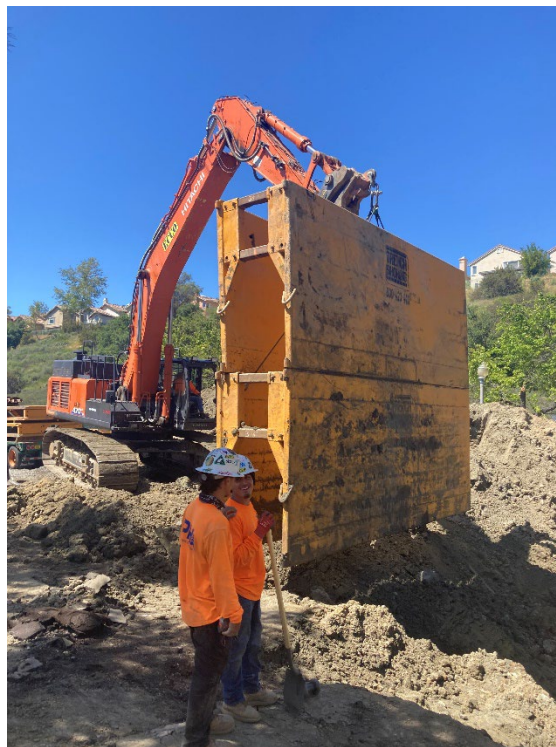
Removal of conventional, trench box shoring materials.
