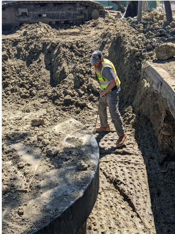
GMU Soil Technician field observing and assessing backfill and compaction efforts.
