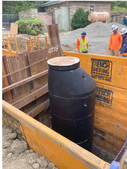
Continued and completed installation of Diversion Mahole.
