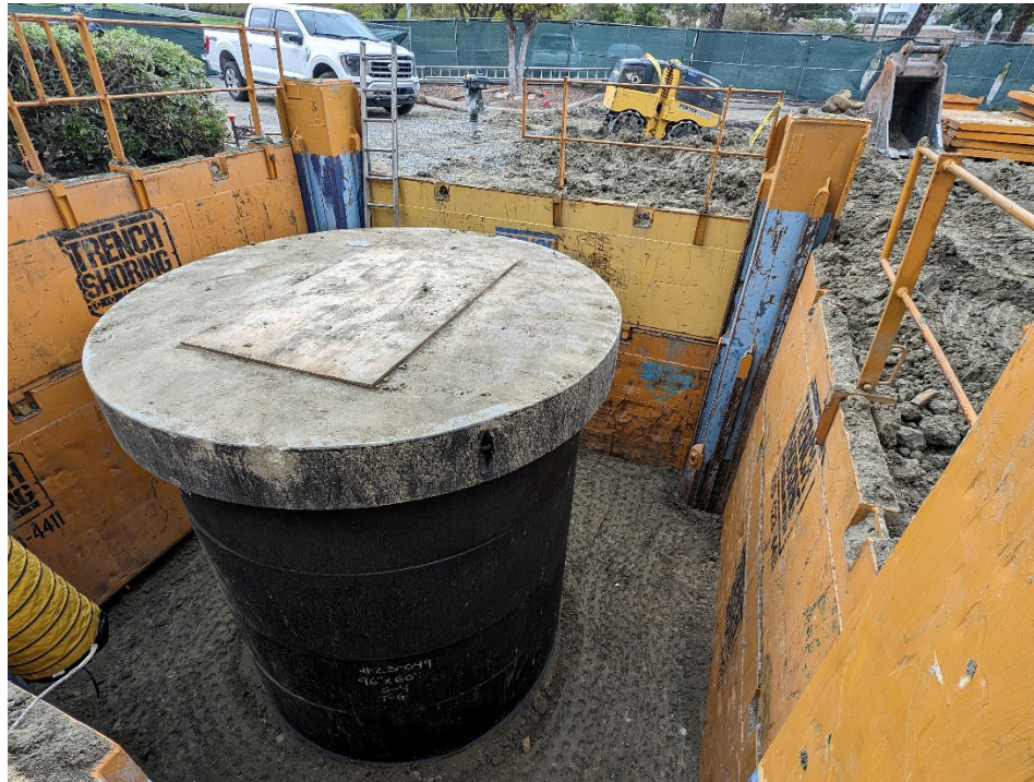
Continued to backfill and compact materials towards grade.
