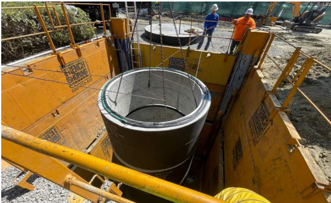
Furnish and Install Pre-Cast Shaft of Bypass Wet Well
