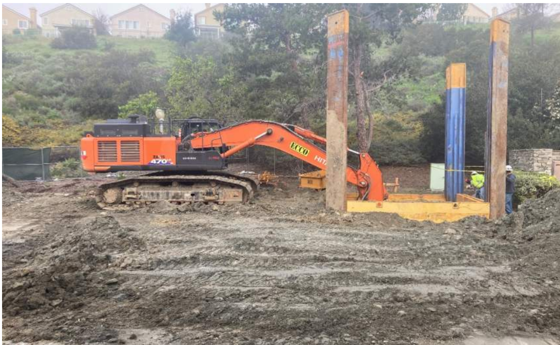
Continued Excavation with 100,000 Pound Excavator
