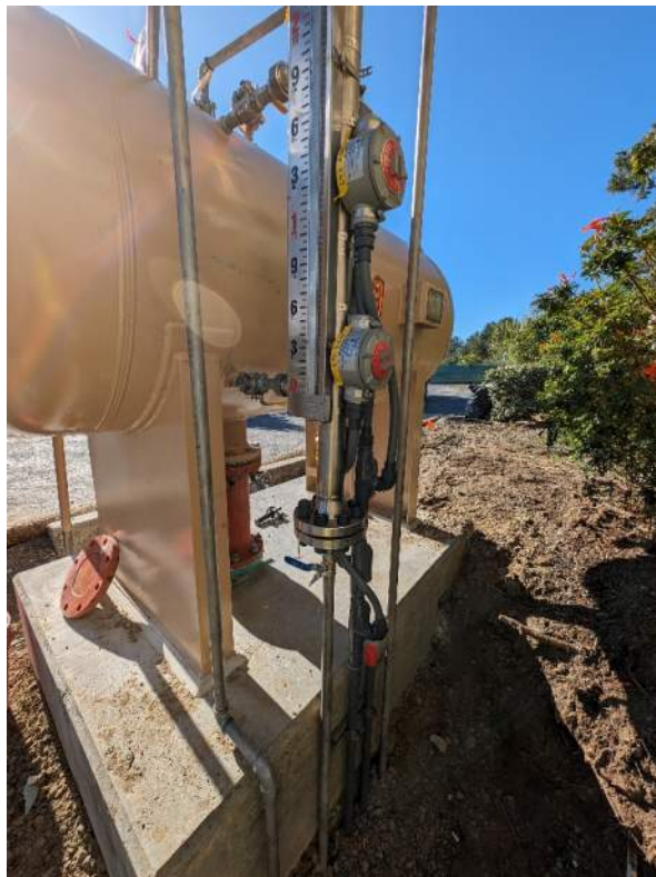
Level Controller, Gauges, and Sensors installed on the Surge Tank
