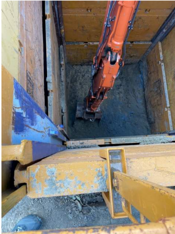
Bottom of Excavation and Placement of Rock Base
