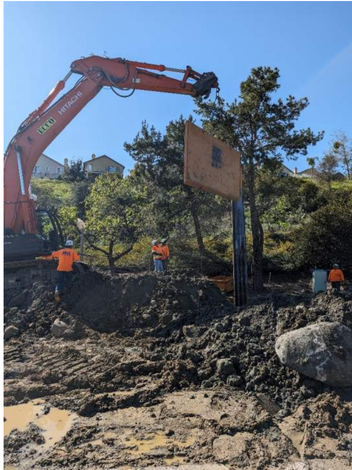
Excavation and Installation of Slide Rail Shoring Components
