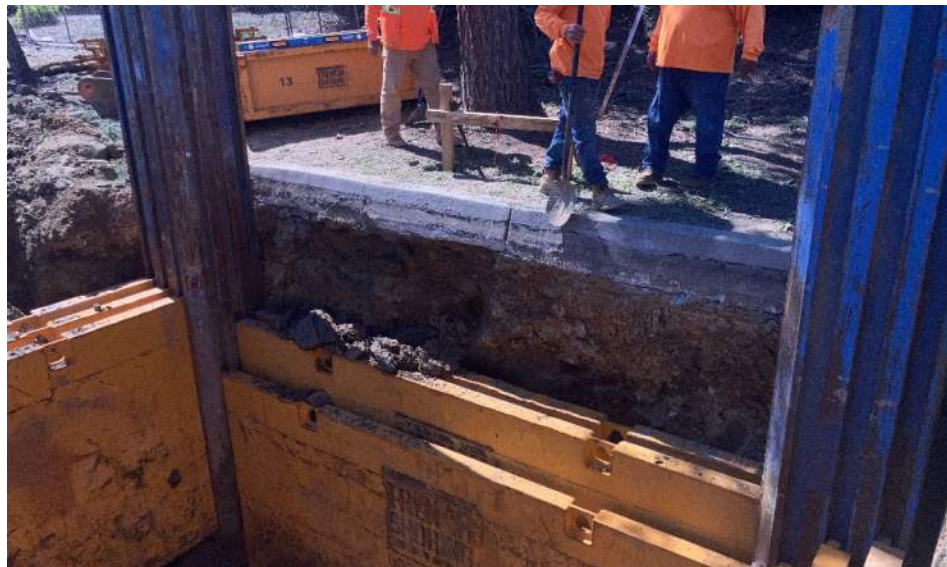
Slide Rail Shoring System Installation
