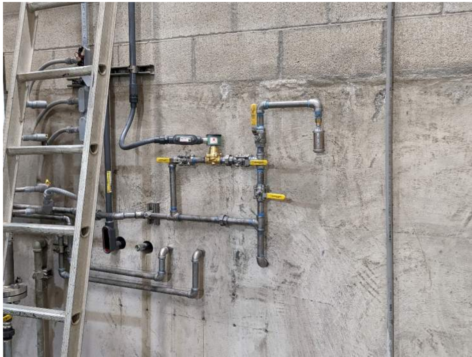
Completed Mechanical Piping for Surge Tank
