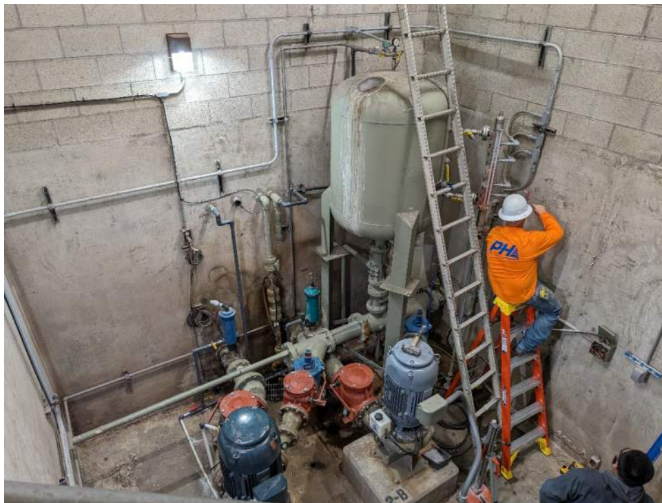
Installation of mechanical piping in Dry Pit of Existing Lift Station
