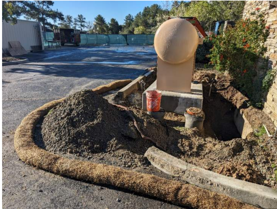
Installation of mechanical piping in from Surge Tank at exterior of Existing Lift Station
