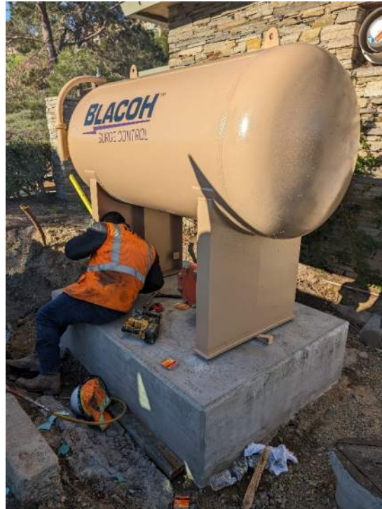
Continued installation of the Surge Tank
