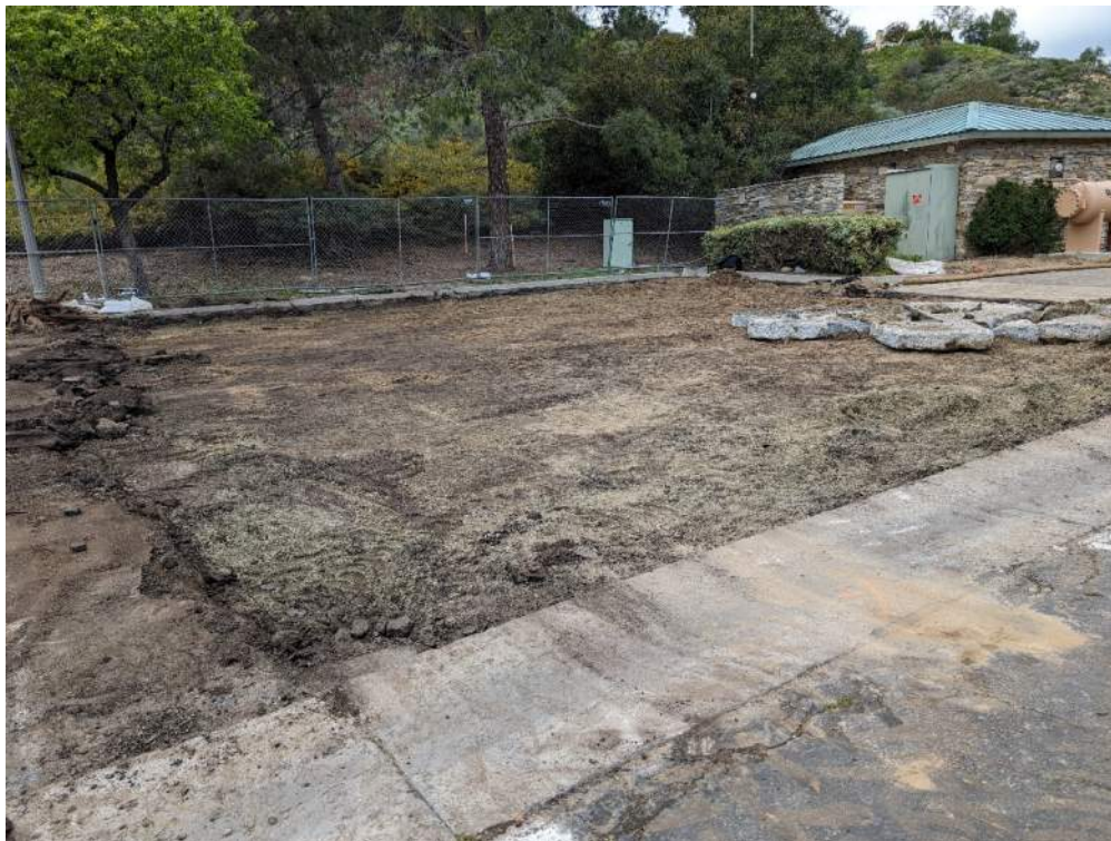
Asphalt Pavement Removals in Preparation of Bypass Wet Well Excavation
