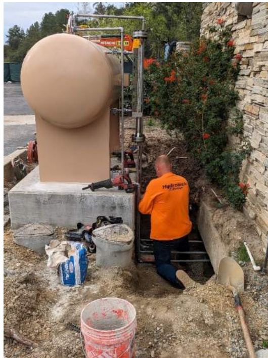
Hydrotech Electric installing instruments and conduits to supply Surge Tank
