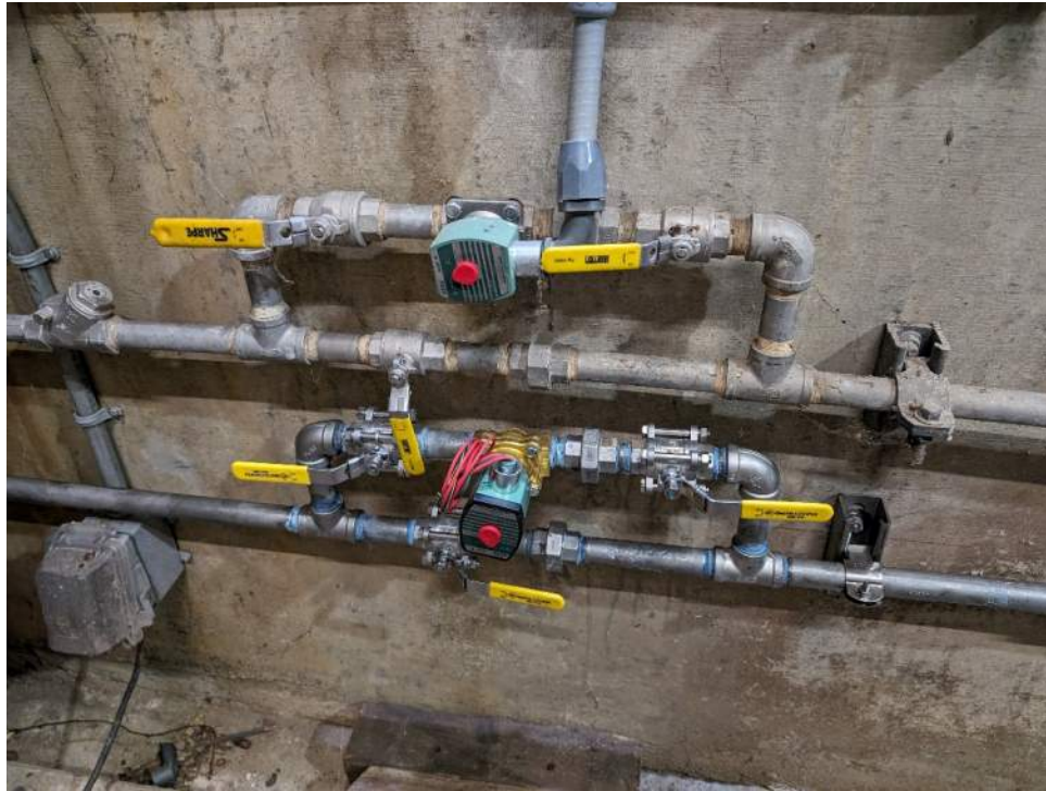
Mechanical Piping and Solenoids at Air Compressor
