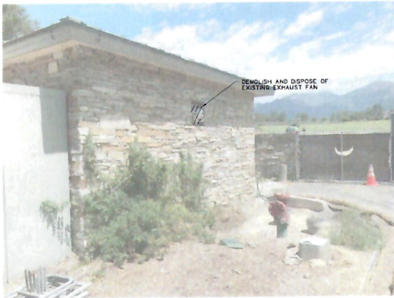
DEMOLITION DETAIL 2 NOT TO SCALE
