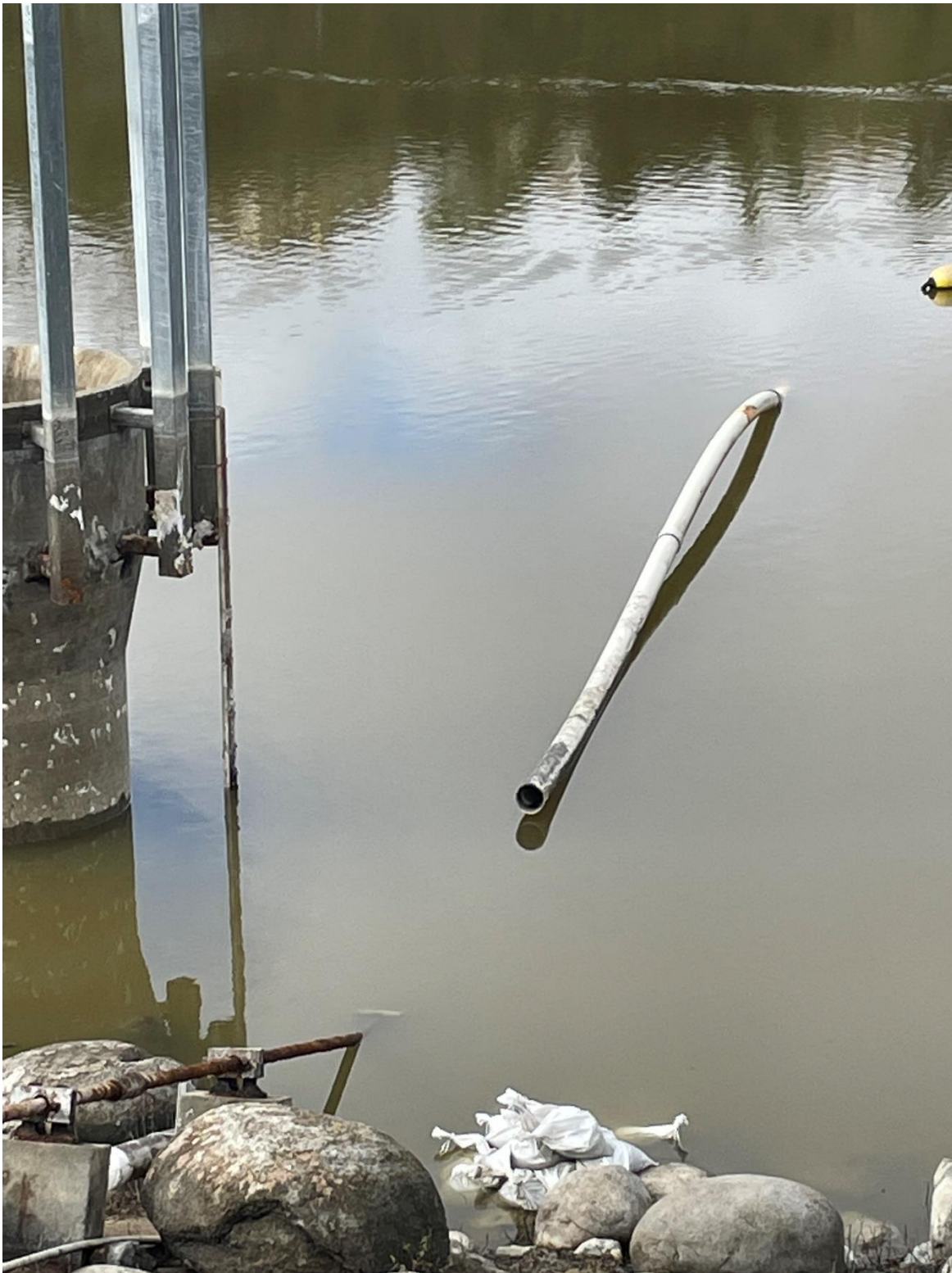
Photo of Dove Lake and PVC Vent Pipe Separation, January 4, 2023
