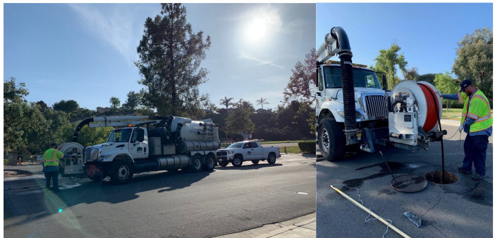
Operations staff cleaning the District’s sewer system
