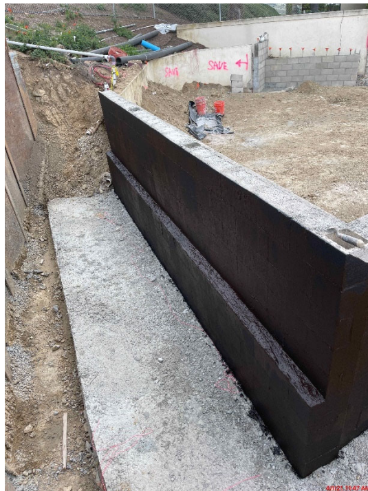
Waterproof Coating for new Retaining Wall
