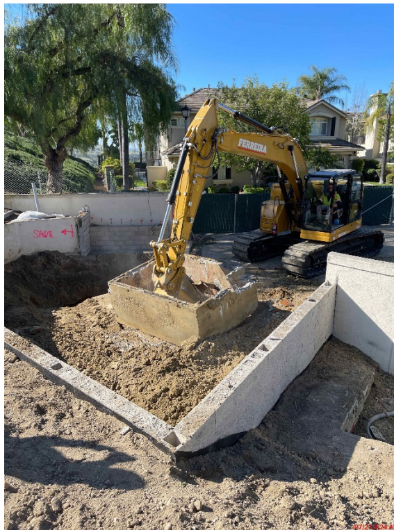
Removal and demolish Existing Wet Well
