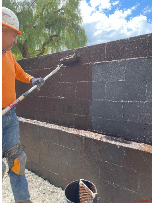
Waterproof Coating for new Retaining Wall
