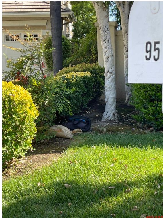
Vibration Monitoring Devices for residents of 93 & 95 Bell Canyon Drive during Demolition Efforts
