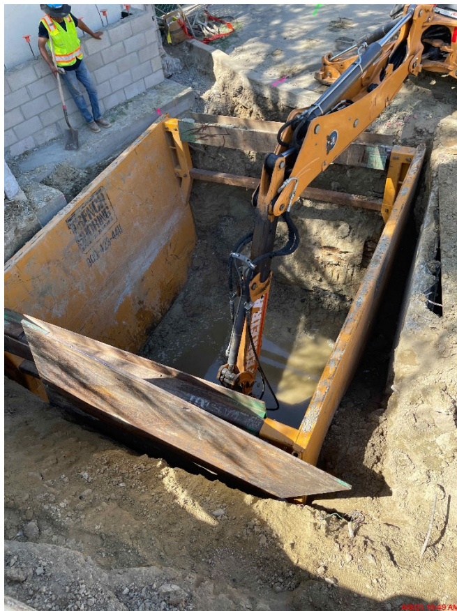
Excavate to bottom of Wet Well
