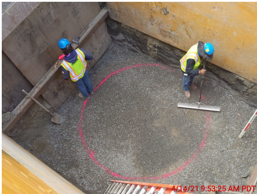
Setting Wet Well
