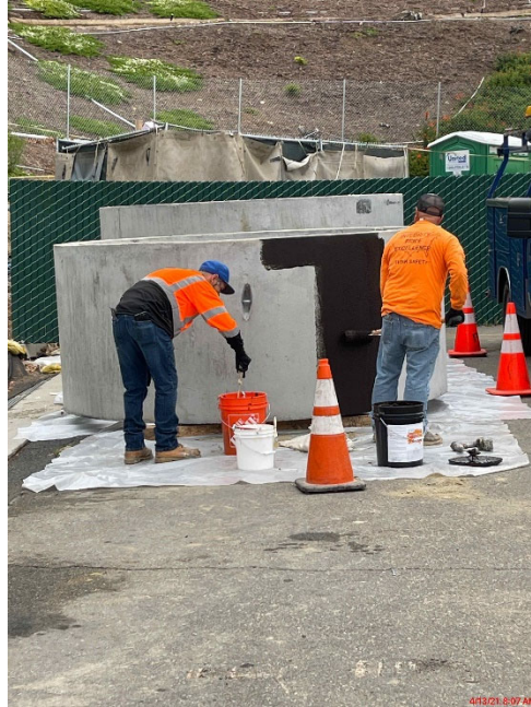
Waterproof Coating Sections of Wet Well
