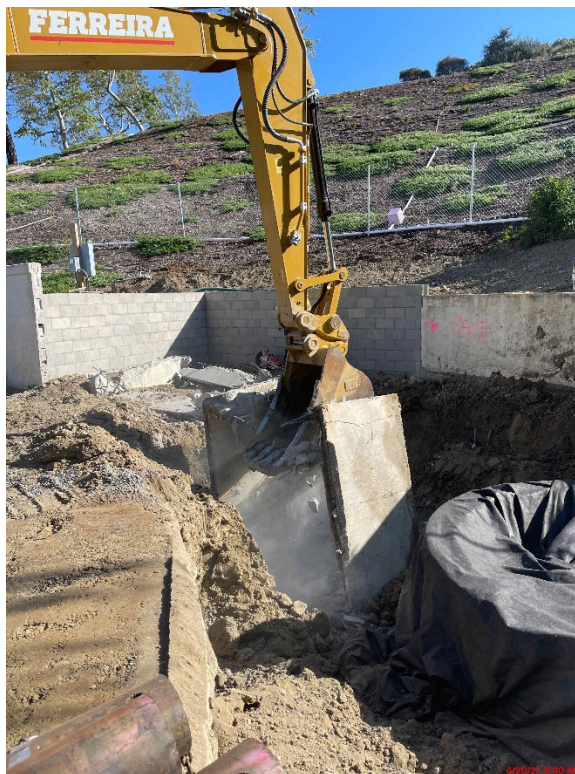
Demolish Existing Dry Well
