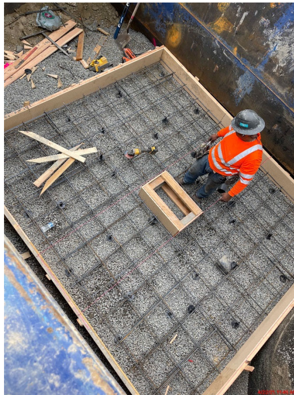
Form and reinforce Dry Well Concrete Slab
