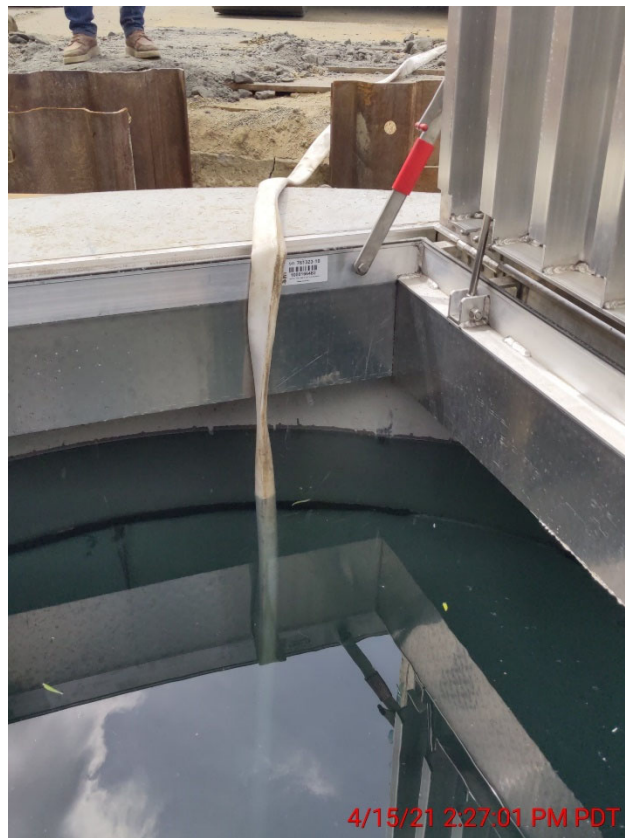
Leakage Test performed and accepted
