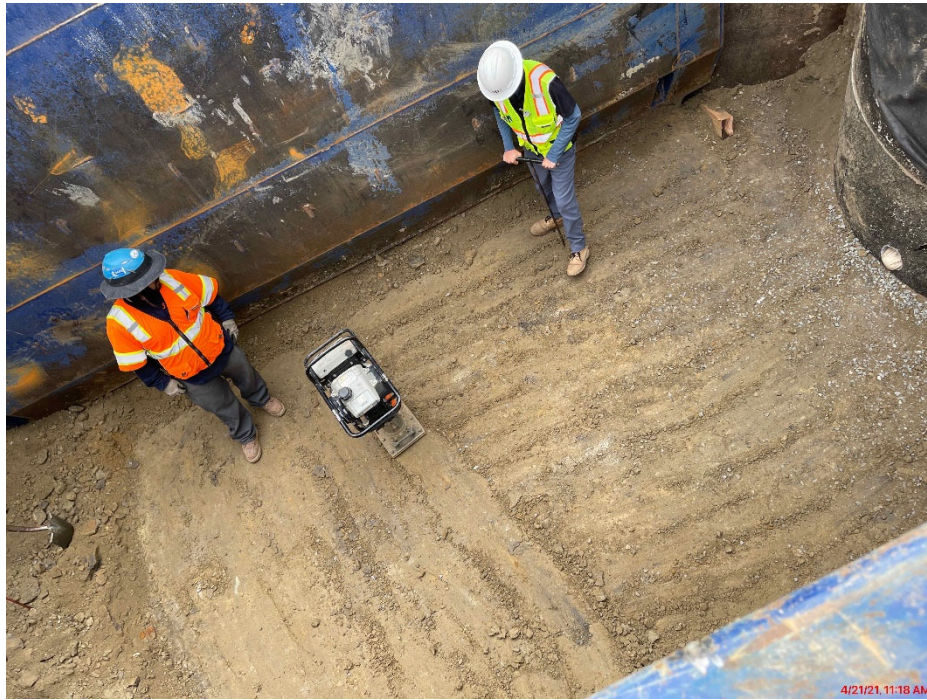
GMU Certified Bottom of Dry Well
