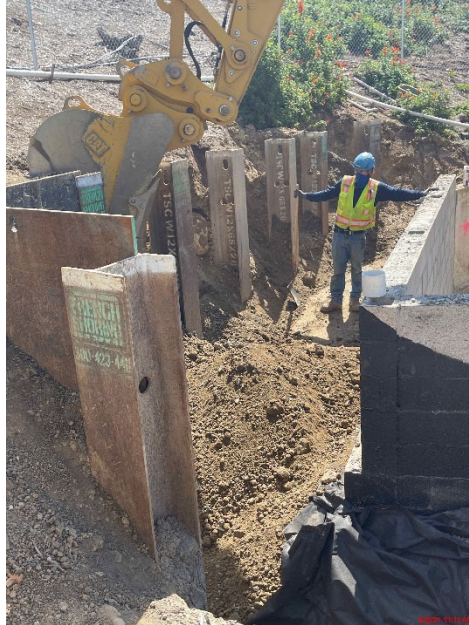
Shoring Removal after Retaining Wall is constructed
