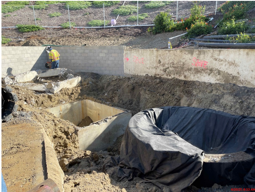
Removal of Existing Dry Well
