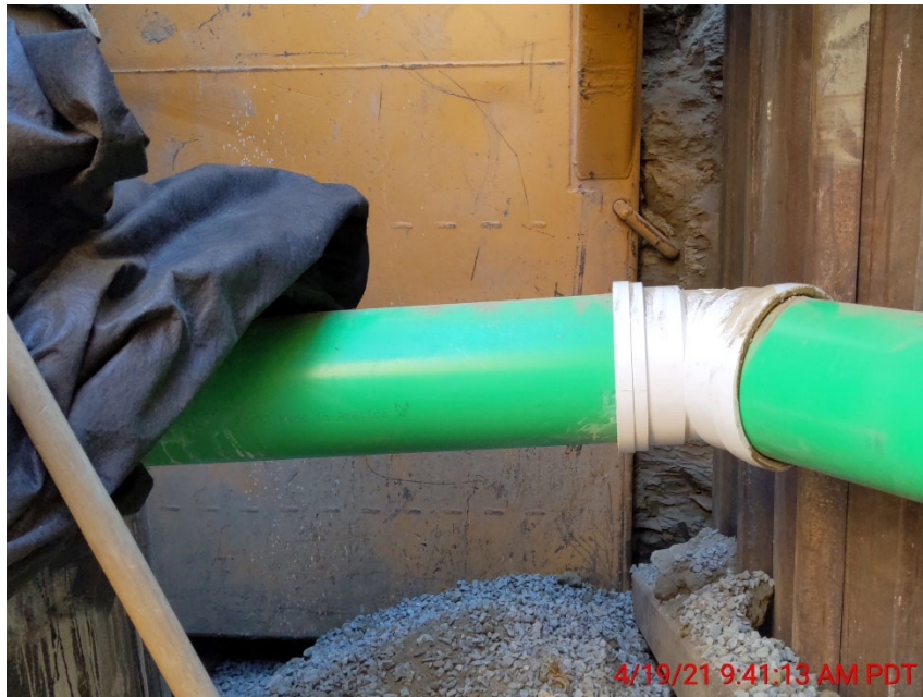
New 8-inch Sewer Line Extension and Connection to Existing Sewer Line
