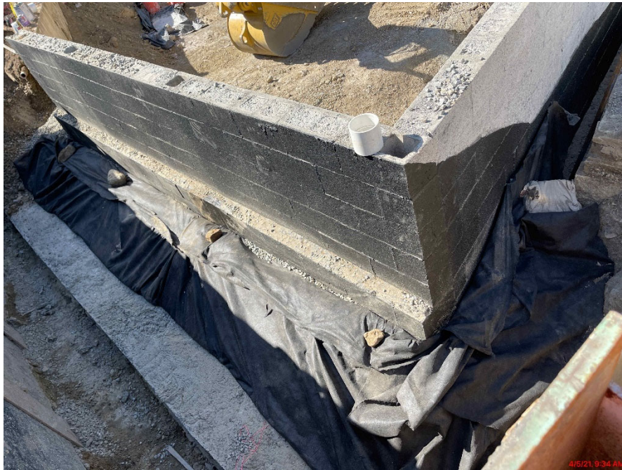
Preparation for Subdrain System
