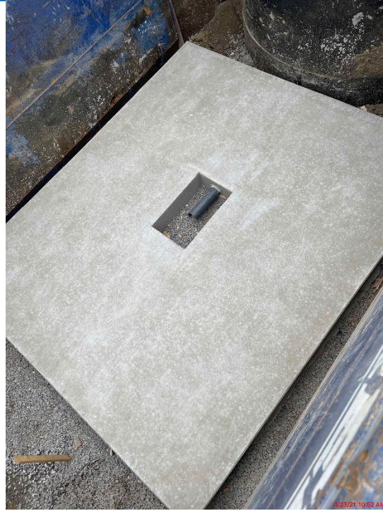
Concrete Slab for Dry Well
