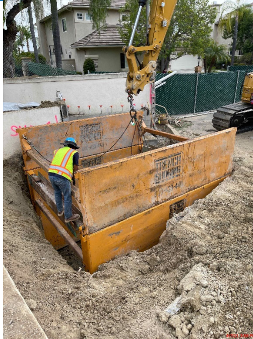
Excavate and place Shoring for new, circular Wet Well
