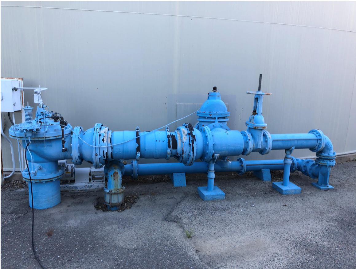
Photo 1 – Existing Reservoir No. 1 Inlet Piping Modification
